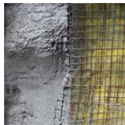
Rockwork Structural Coat
